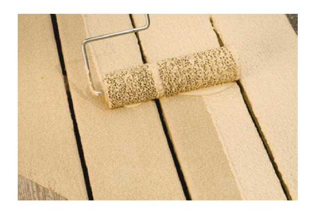
**APPLY THE SECOND COAT.** Allow final coat to dry at least 8 hours before foot traffic and 24 hours before replacing furniture or heavy objects. Drying time may vary due to weather conditions. Deck Restore™ cures to a hardened finish in approximately 3 weeks. Touch ups and partial recoats are easy for repairs and blending to create and maintain the ideal finish.
