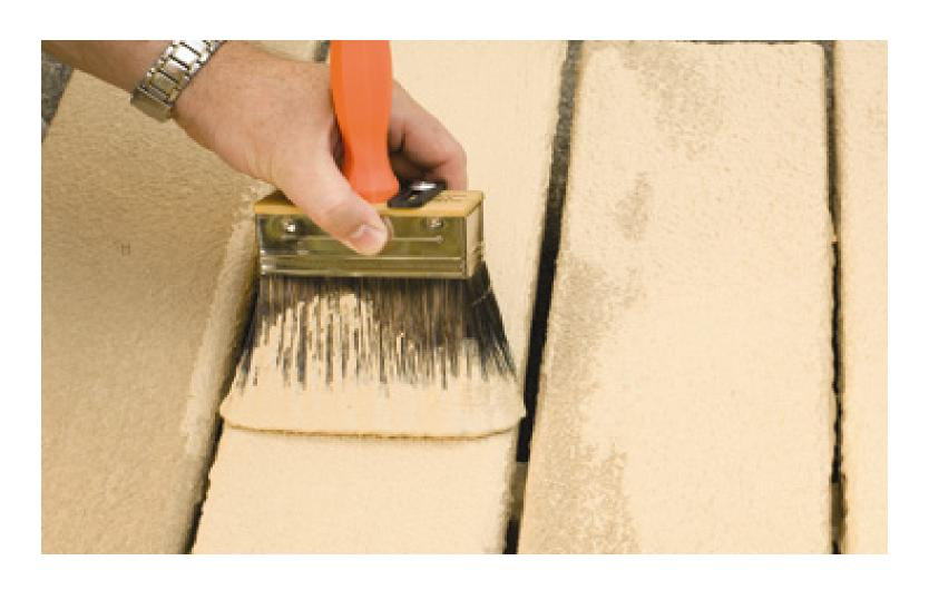
A brush may be used to skim the rolled application in a back brushing motion in one direction. This will provide a smoother textured look. Use care not remove any material already in place by applying too much pressure.
