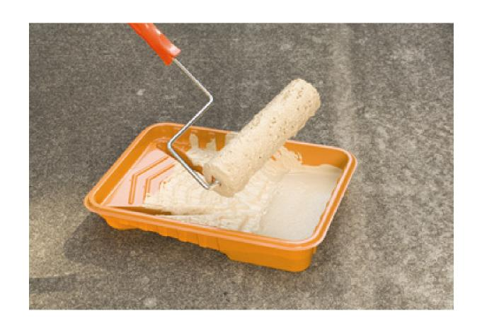
Saturate the Restore Roller™ roller cover in the coating by rolling back and forth in the tray. A fully loaded roller will cover a spread area of approximately 5-7 square feet.
