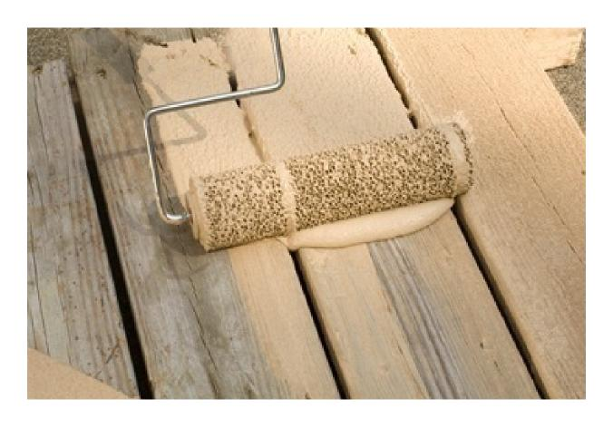
APPLY THE FIRST COAT by using slight pressure to disperse the coating evenly through the honey comb webbing. The two gallon kit will cover approximately 100 square feet for the first coat application.
