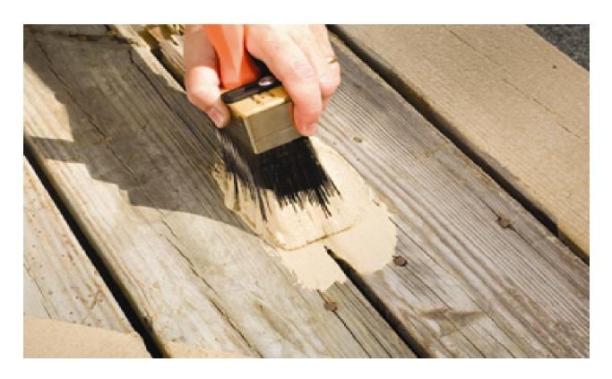
Deck Restore™ will fill nail holes and cracks up a ¼". Fill these damaged areas with a heavily loaded roller or brush by dabbing until the gaps or cracks are filled.
