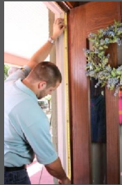
Measure height of door
