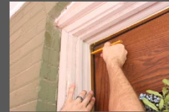
Mark holes through seal
